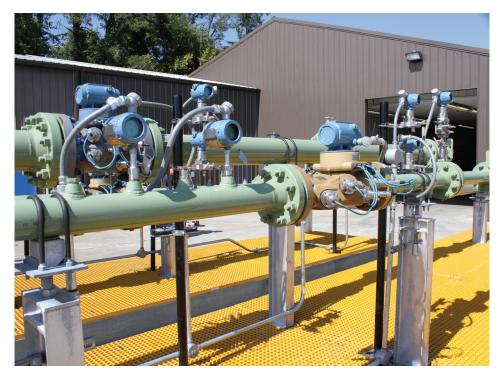
Modular Sample Control Panel and a Mustang Moisture Analyzer System which provides an Analytically Accurate® sample to the GC for gas composition analysis.
